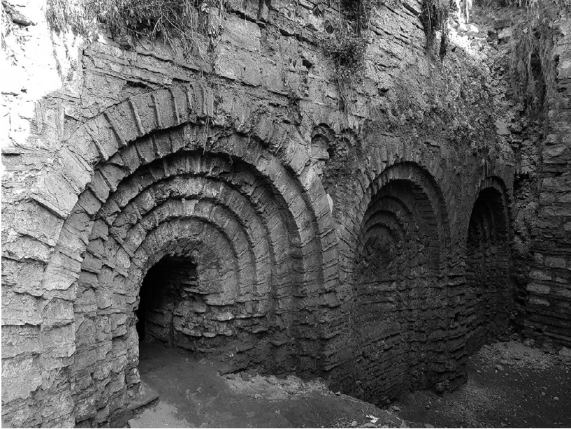
4.5 Fountain house near Unkapani, Istanbul, middle Byzantine period. (Courtesy of Kerim Altuğ)
